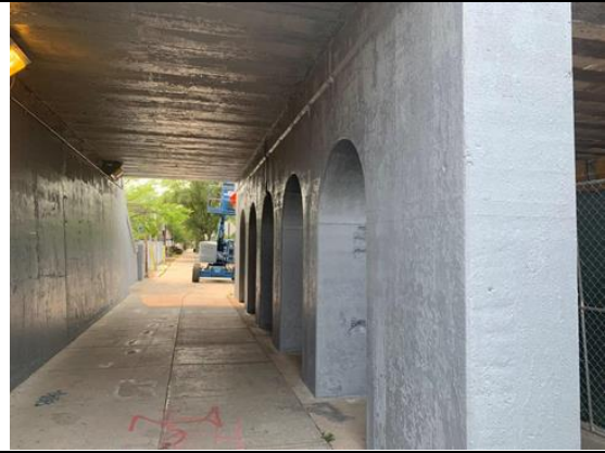
Chicago 63rd Street Viaduct, fully encapsulated after Dan's Community Project
